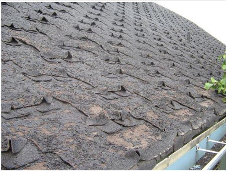
**“As your composition shingle roof ages you'll see bits of roof material and granules accumulating in the driveway.”**
